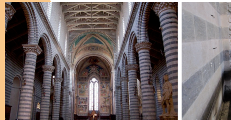
Fig. 4.17 - Left: inside of the cathedral of Orvieto showing the balcony along the aisle walls, between the windows and the arches. Right: evidence of two sensors, barely visible as a dark bar on the white stripe of the wall.
