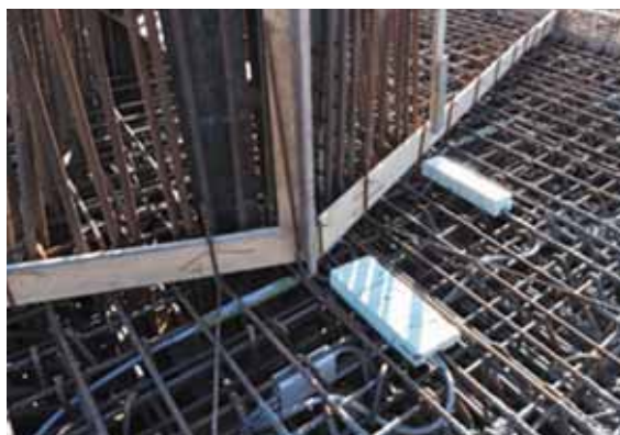
Figure 89 – a) Cross section view drawing of one pavilion and a picture of the structure soon after completion of the dome frame. Phases of the installation of the FBG sensors on various structural components during construction works b)
