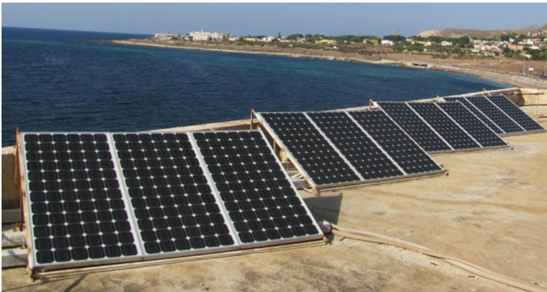
Figura 1. Campo FV in Si-m.
