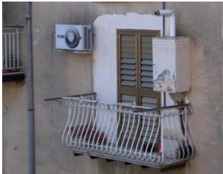
Figure 2: Typical individual heating and cooling systems in the southern Italy (Sven Werner) [10].
