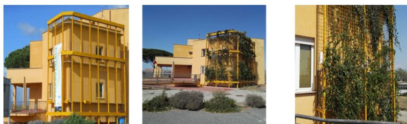
Figure 1. Green wall prototype installed at the ENEA Casaccia Centre.
