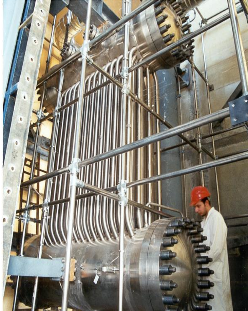
ESBWR Isolation Condenser
