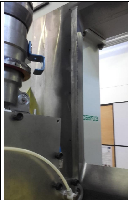
Fig.20 2nd cleaning phase
