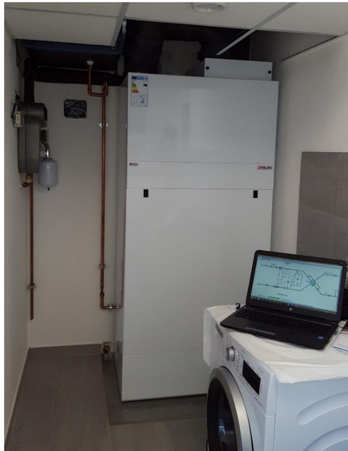
**Figura 4-2** Aggregato compatto Nilan Compact P
