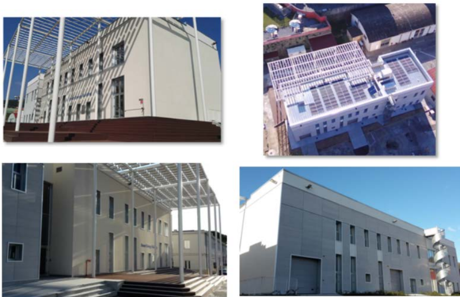
Figura 3 – Lo Smart Energy Building (SEB) del campus
