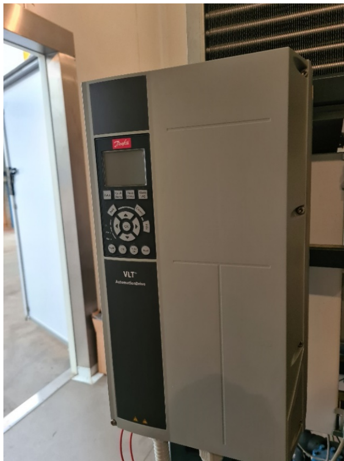
Figura 19: Inverter Danfoss VLT Automation Drive FC-302P4K0T5 montato sul Prototipo #1.
