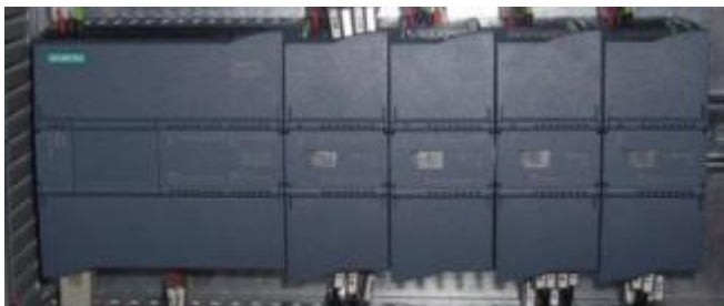
Figura 31. PLC Siemens S7-1200
