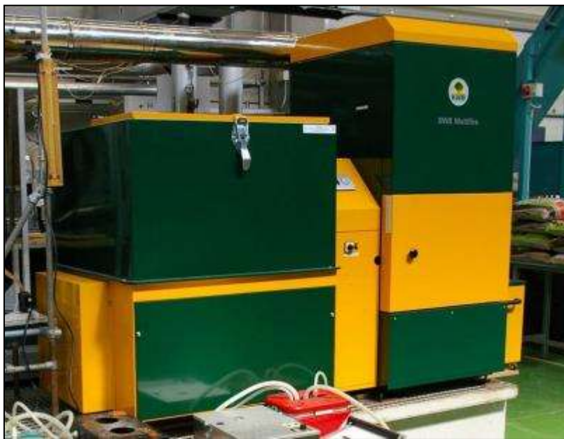
Figura 1. Caldaia a biomassa KWB Multifire USV V 30
