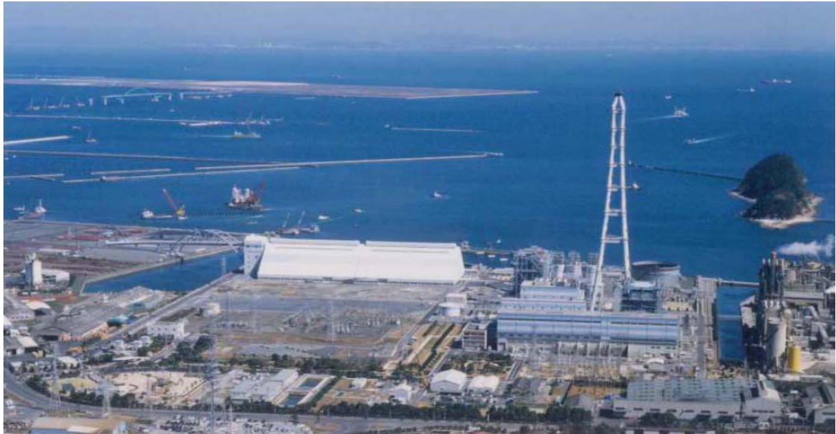
Figura 4.12. Impianto PFBC Karita Therma Power Station 32 .
