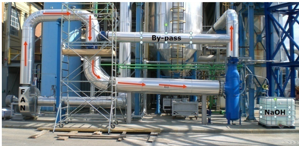
Figure 4 Condenser and neutralization system
