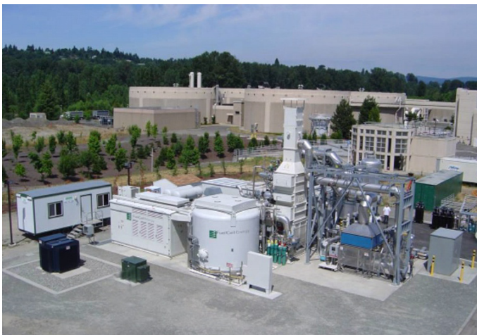
Figure 2. King County Power Plant (courtesy of FCE)
