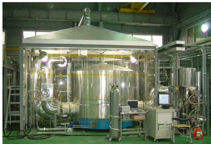
Figure 8. A 25 kW-class Internal Reforming MCFC stack at DHI
