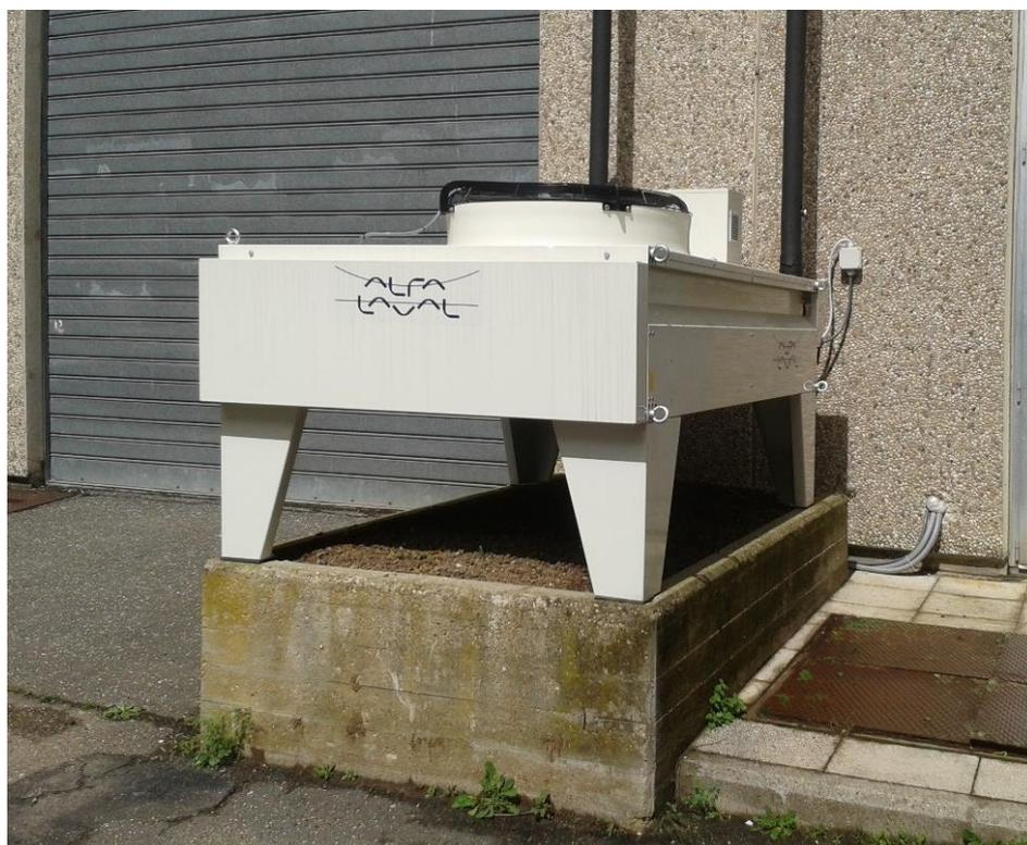
Figura 15. Dry Cooler Alfa Laval
