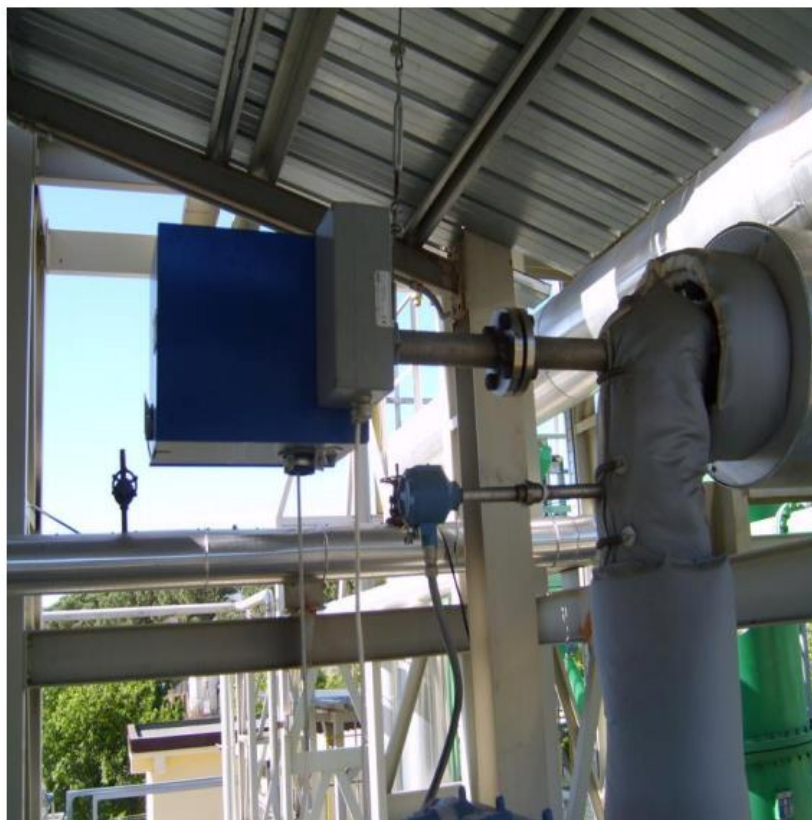
Figure 1. Photograph of sampling probe in sampling point V2
