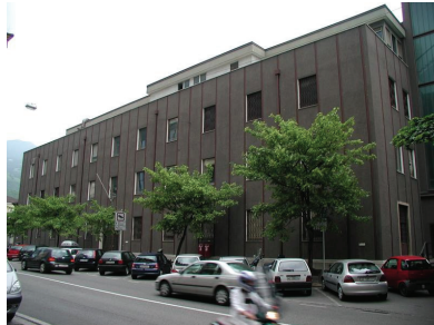
Fig.5: View of the building before retrofit
