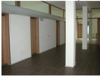
Fig.8: View of the interior of the building after retrofit.
