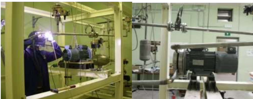
Figure 4 - installation of the pump and final configuration
