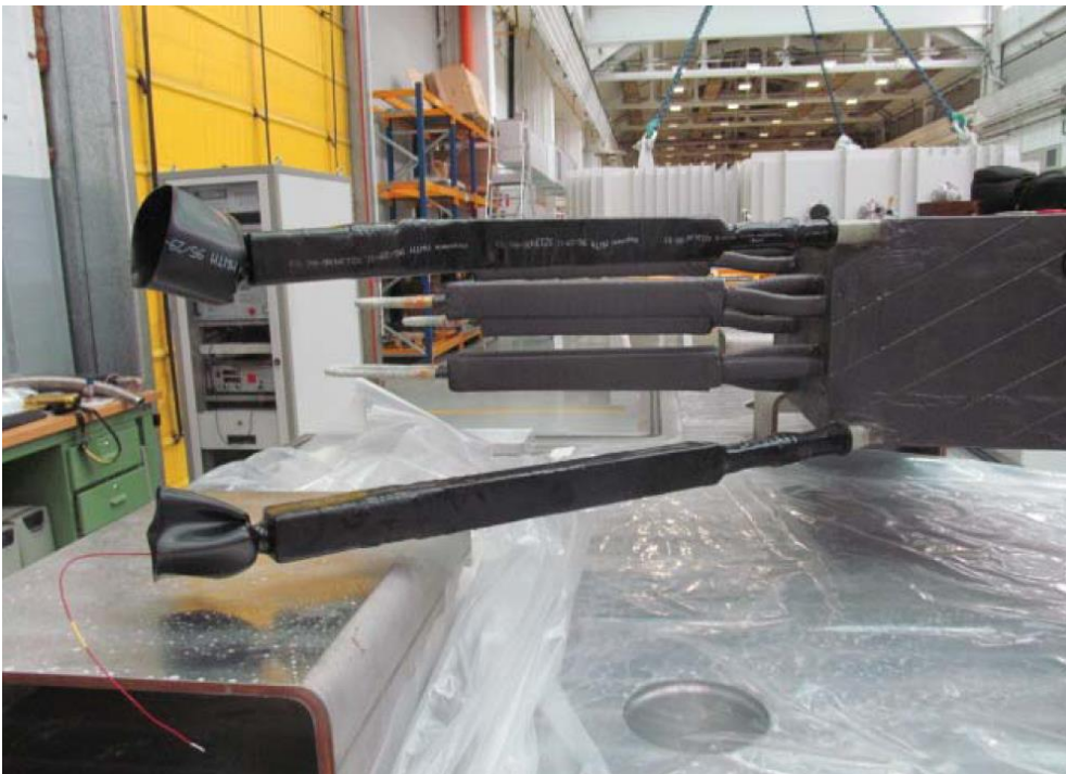
Fig.15 – Temporary insulation on terminations needed to carry out Paschen test.
