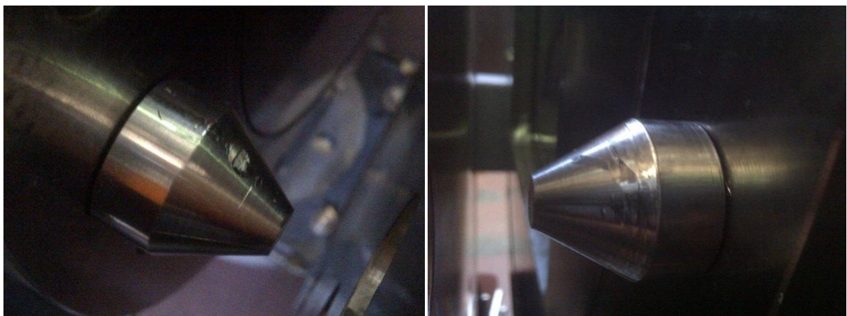
Fig. 30 Status of the dowel pins of the flange of the beam
