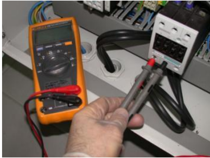
Figure 22: Check for the electrical continuity of the heating resistance
