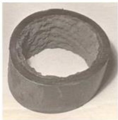
Slag in pipeline
