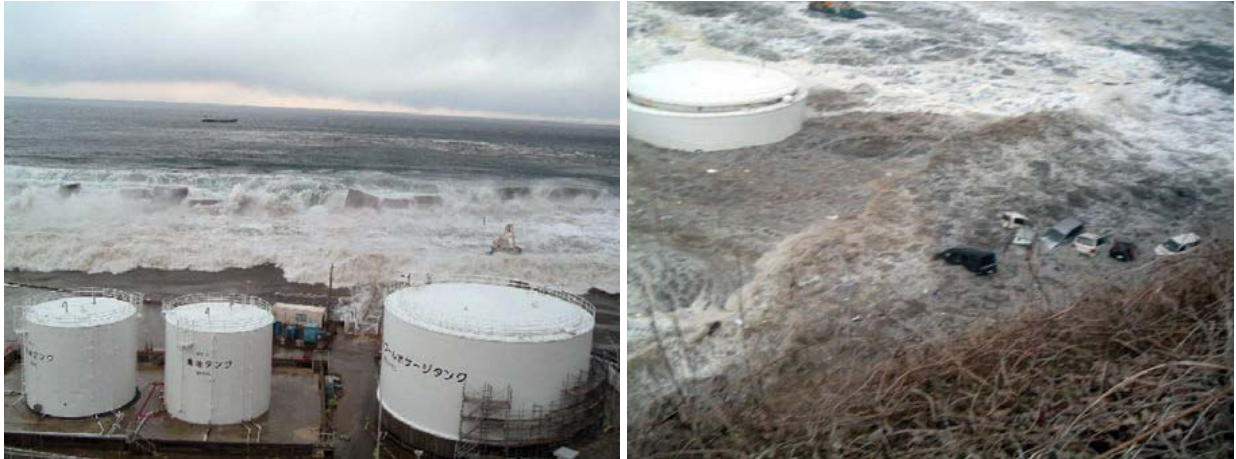
Figure 21 - Tsunami waves impinging on the 6 m protective wall of the nuclear plant
