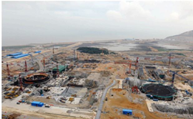
Taishan units 1&2 overview (April 2010) scope
