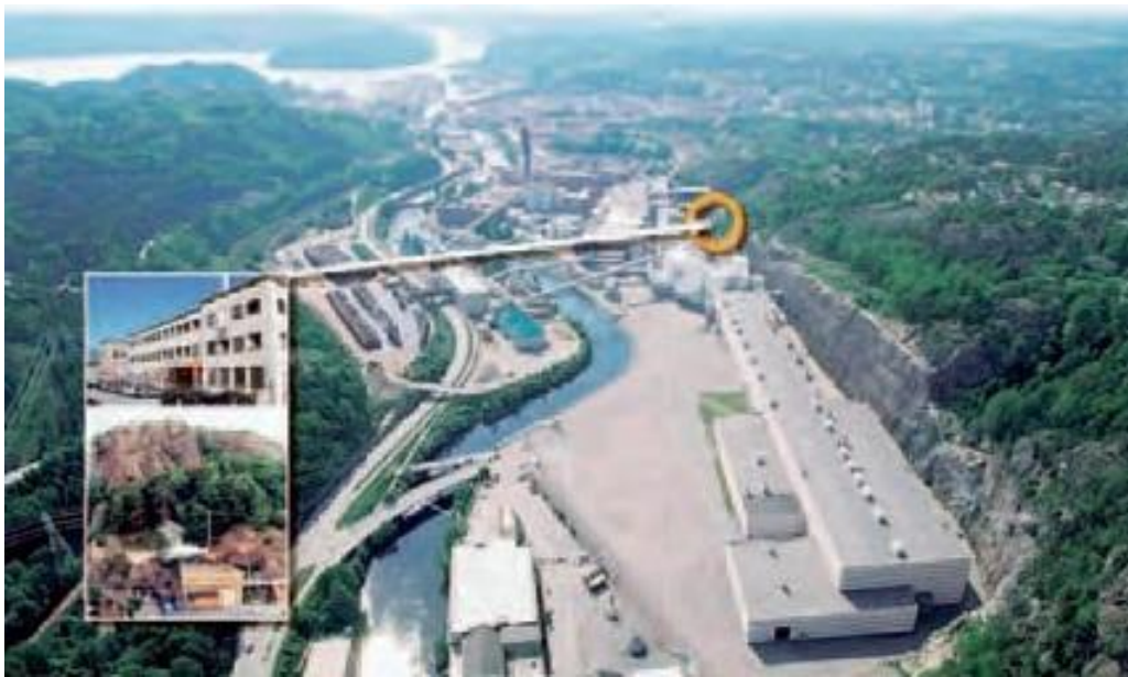
Fig. 1. Site area of the BHWR in Halden.
