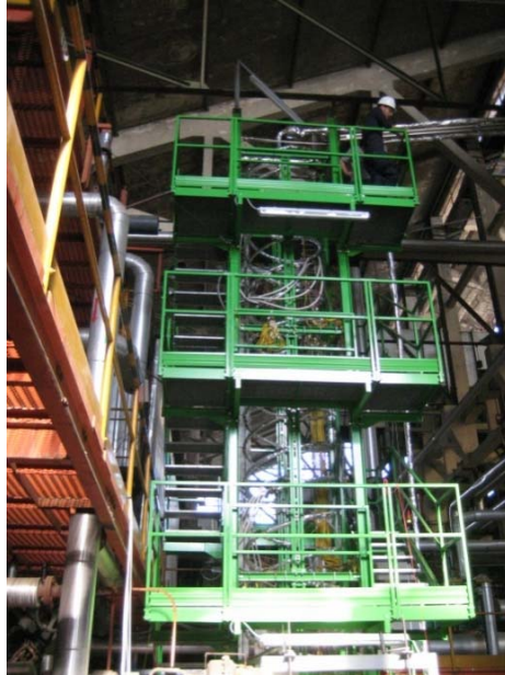
Fig. 2. Global view of the facility test section.
