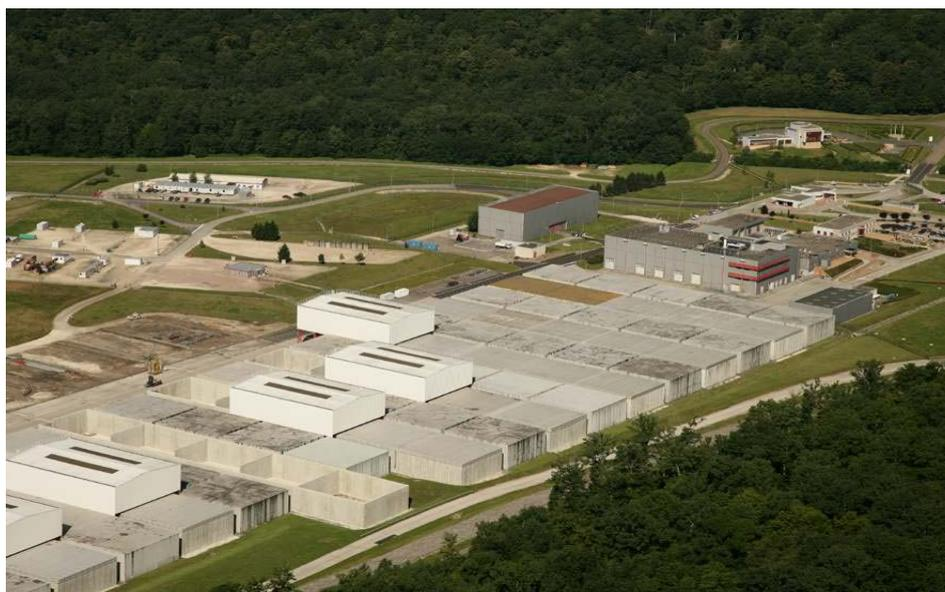
Figure 6: Disposal vaults and mobile roofs .
