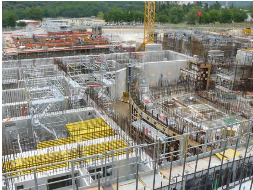
Figure 5: JHR construction site in 2011, nuclear auxiliaries building.
