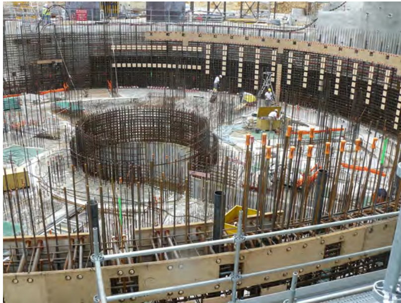
Figure 4: JHR construction site in 2011, reactor building.
