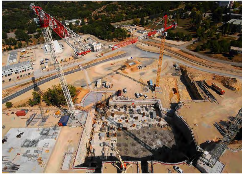
Figure 2: JHR construction site at the end of 2009.
