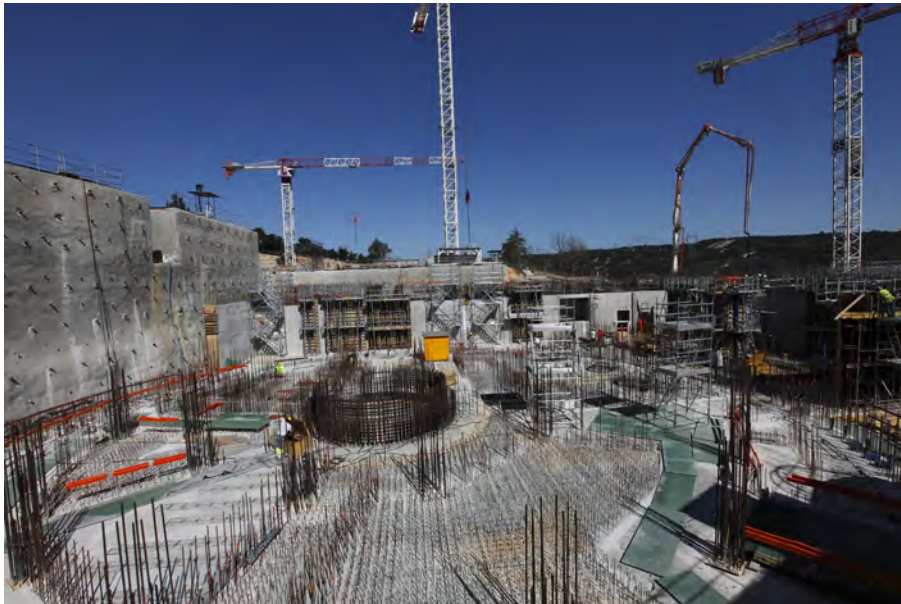
Figure 3: JHR construction site in 2011.
