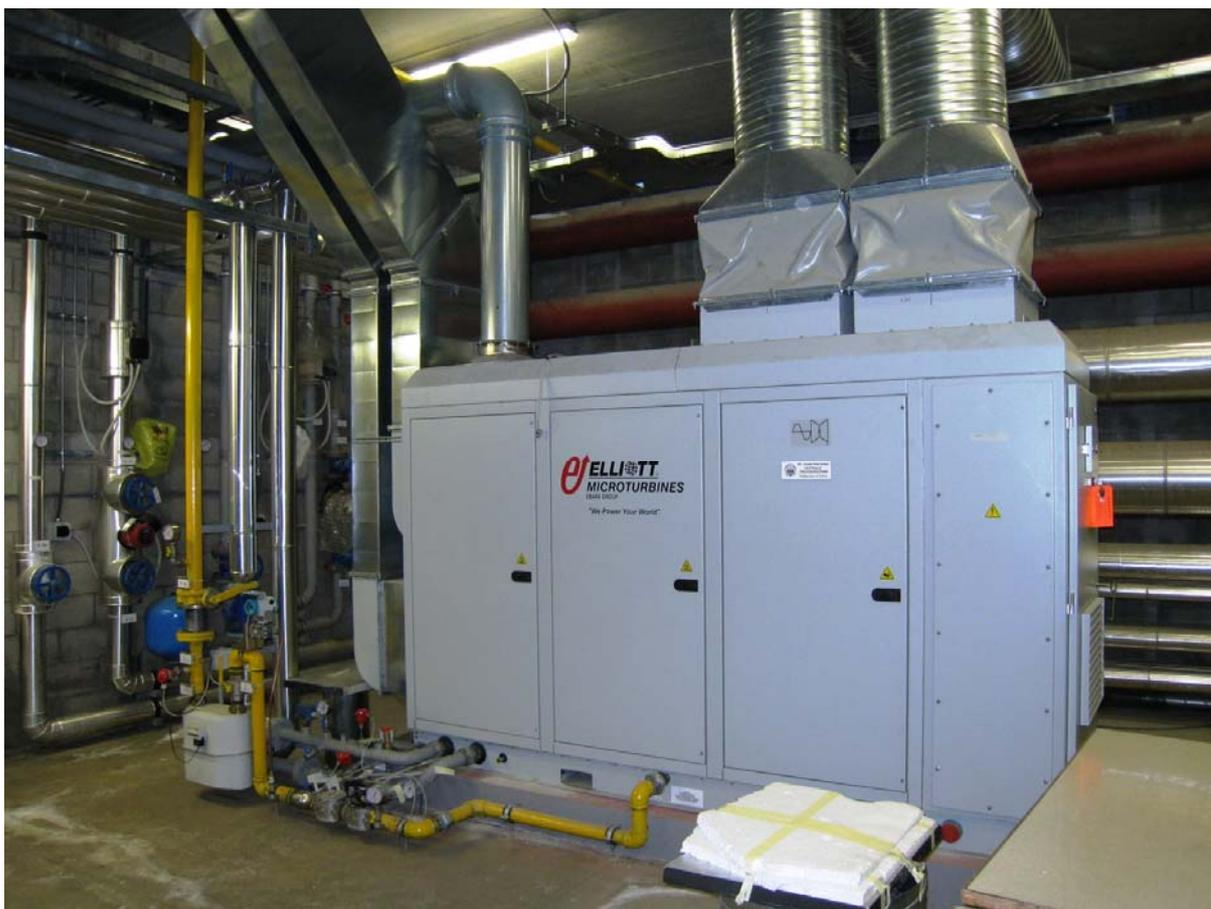
**Figura 3: Microturbina**
